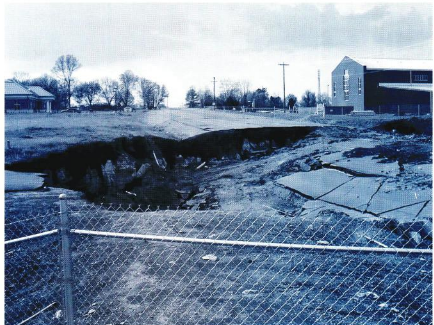
The Dishman Lane sinkhole collapse in Bowling Green, Kentucky.
