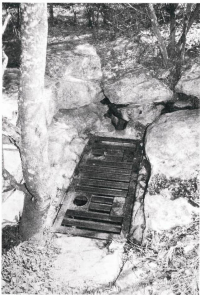
Lakeline Cave, Texas, was gated to protect two endangered invertebrate species. The cave entrance had been burned out by vandals, so a double-lock gate was installed. Note the animal access hole at the far end of the sink for raccoons and mice. Photo by William R. Elliott.
